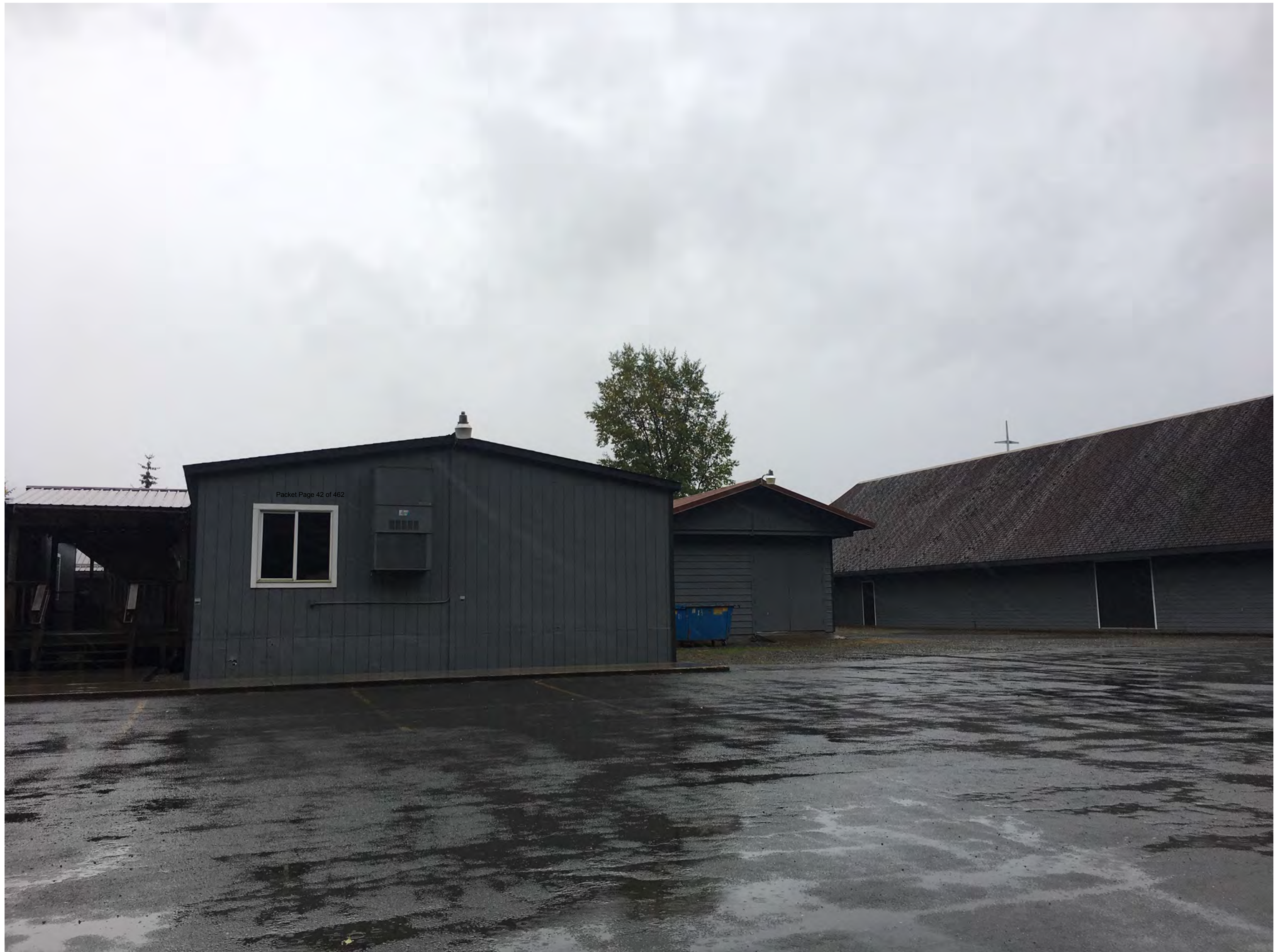
Attachment C - Site Visit Photos
