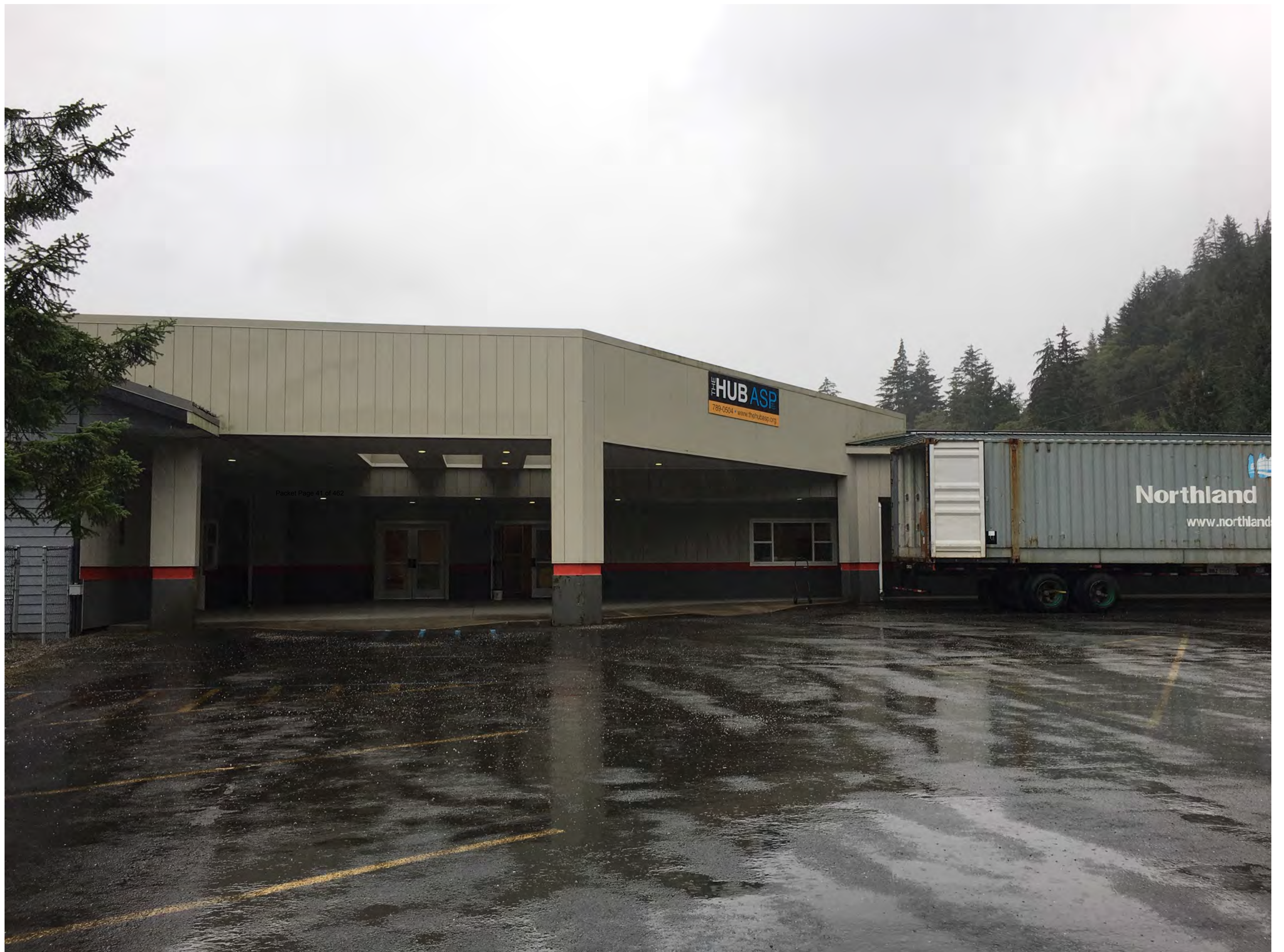
Attachment C - Site Visit Photos
