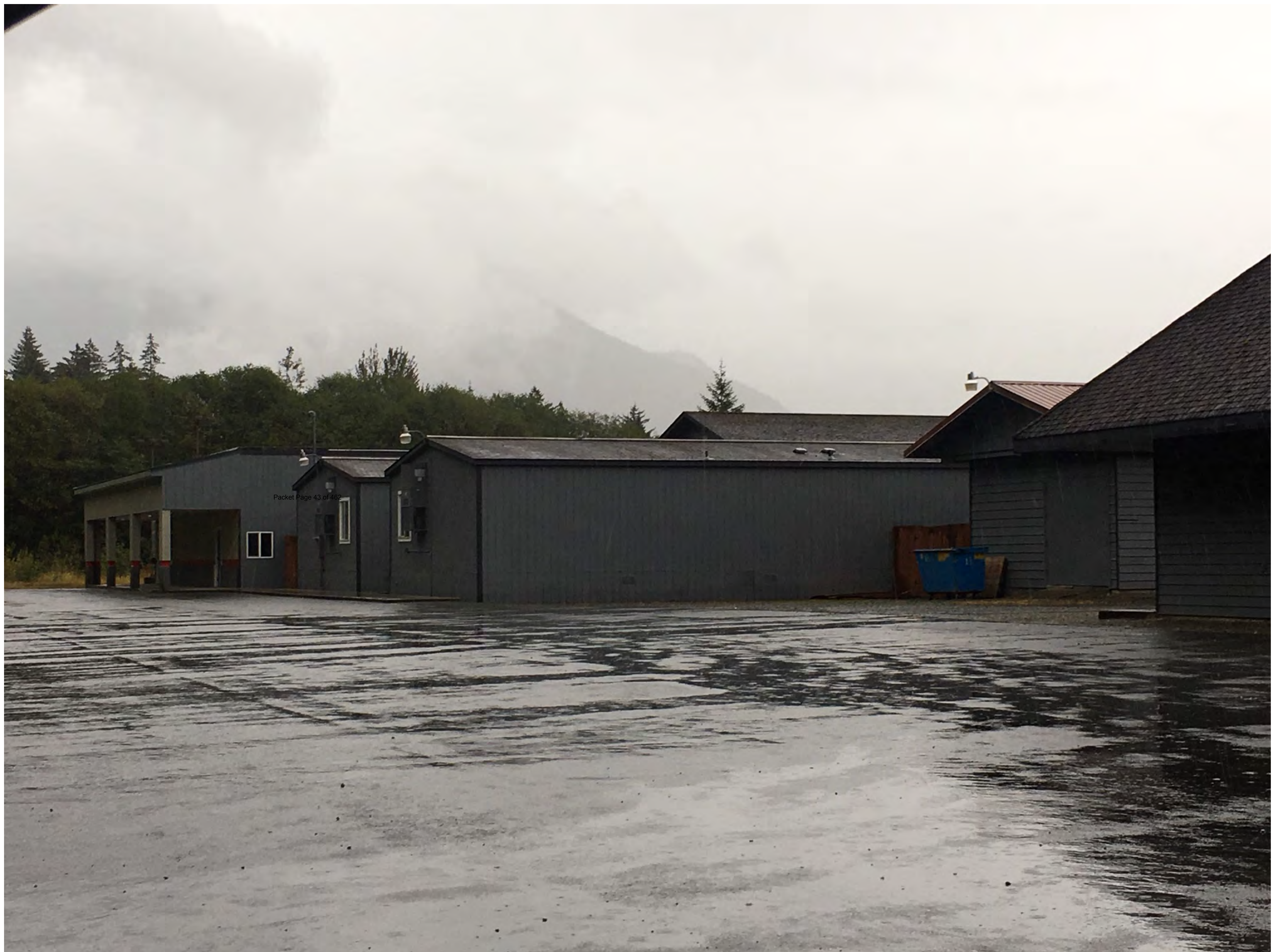
Attachment C - Site Visit Photos
