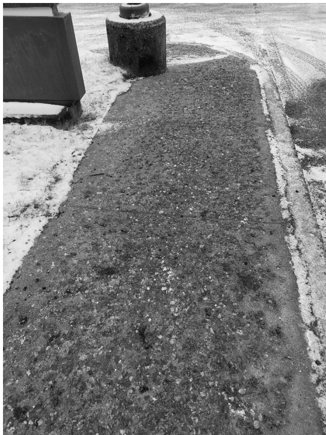
Above: Existing sidewalk in the project area. Note the sidewalk gap between Glacier Highway and Salmon Creek Lane. Below right: Raveling sidewalks.
