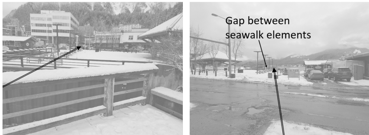
Figure 10 (above): Ground-level views of seawalk connectivity to Seward Street. On the left, standing on the southeast portion of the seawalk looking toward Seward Street (compound arrow). Beyond the railing in the foreground is the gap that will be decked over; the sheet pilings can be seen along the section of the dock near the Warf. On the right, looking toward the waterfront from the pedestrian "lamb chop" refuge island at the intersection of Seward Street and Egan Drive (compound arrow).
