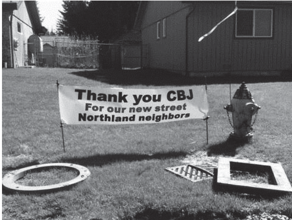
Northland Street Reconstruction
