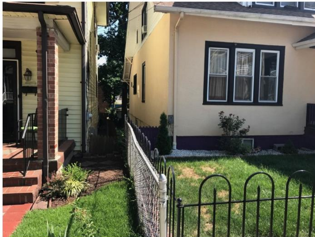
Typical Mount Rainier bungalows on Perry Street. R-55 zoning requires these houses to be 16 feet apart and 25 feet further back. But in reality, they are only 7 feet apart. Image by Brent Rolin.
