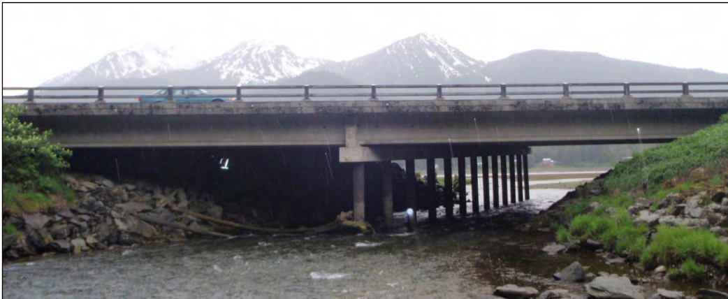
FIGURE 1. Existing Bridge No. 1188 Salmon Creek Bridge.
