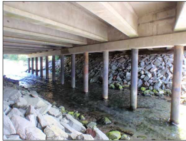
FIGURES 4. Bank treatments under Bridge No. 1188. Photo taken April 6, 2009.
