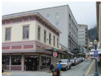
The newly opened heritage coffee shop on the north side has added new vitality to this block.
