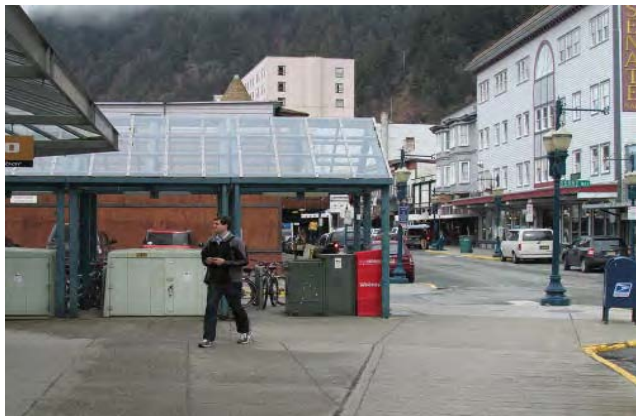
This view looking north on Franklin Street terminates at an existing canopy and electrical switching equipment.
