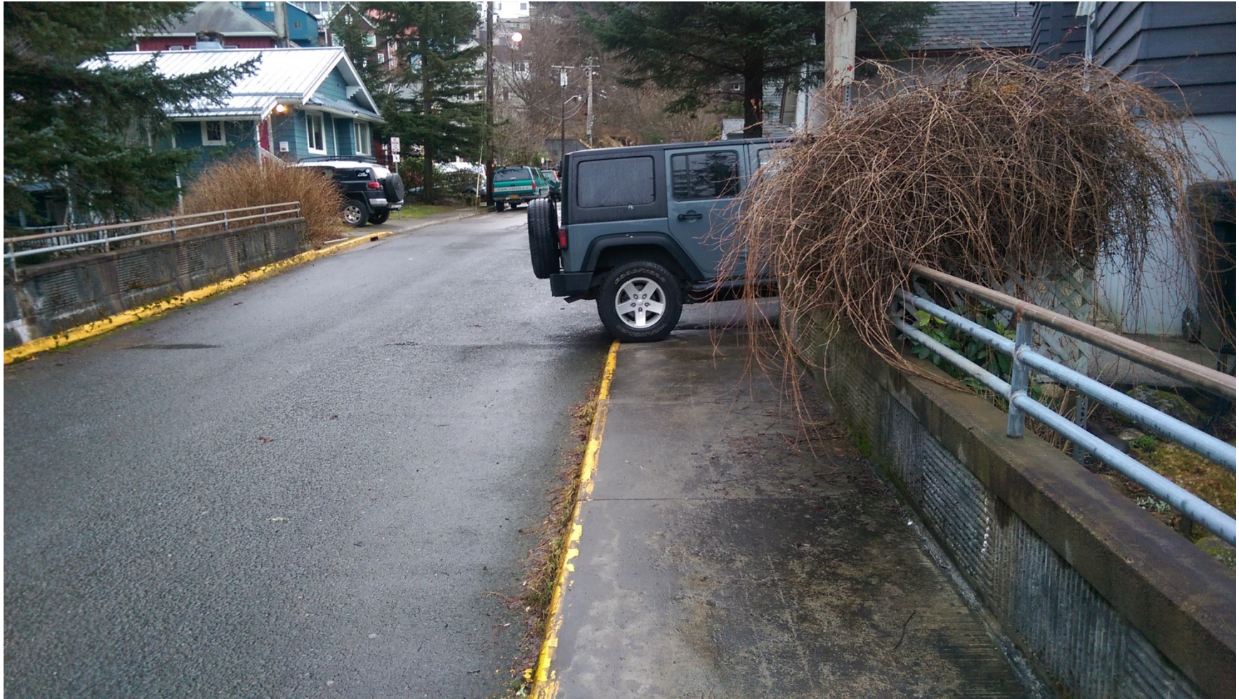
Attachment C2 – W. 8 th Street: Parked car across sidewalk. New sidewalk will continue down this side of W. 8 th Street (See C3). Foliage should be cleared from sidewalk.
