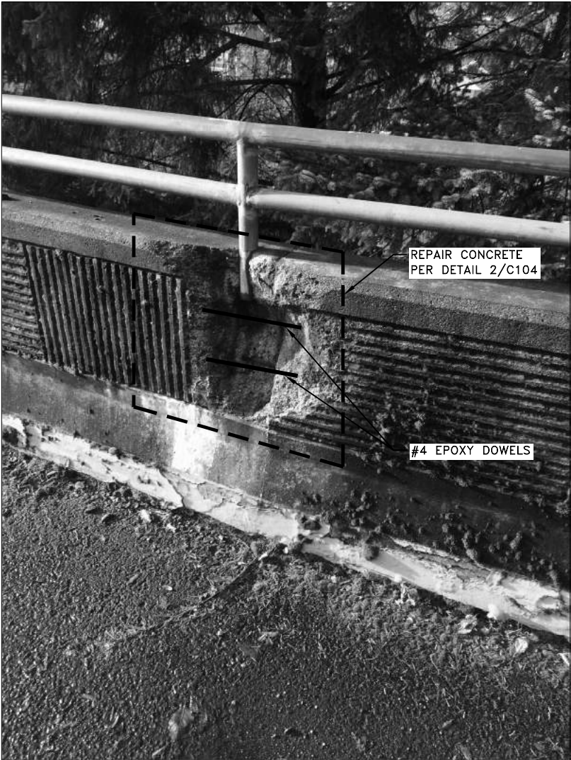
1 PHOTO OF CONCRETE SECTION TO BE REPAIRED N.T.S.
