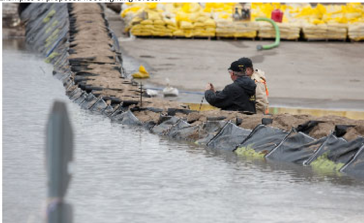
Sand filled Levee System
