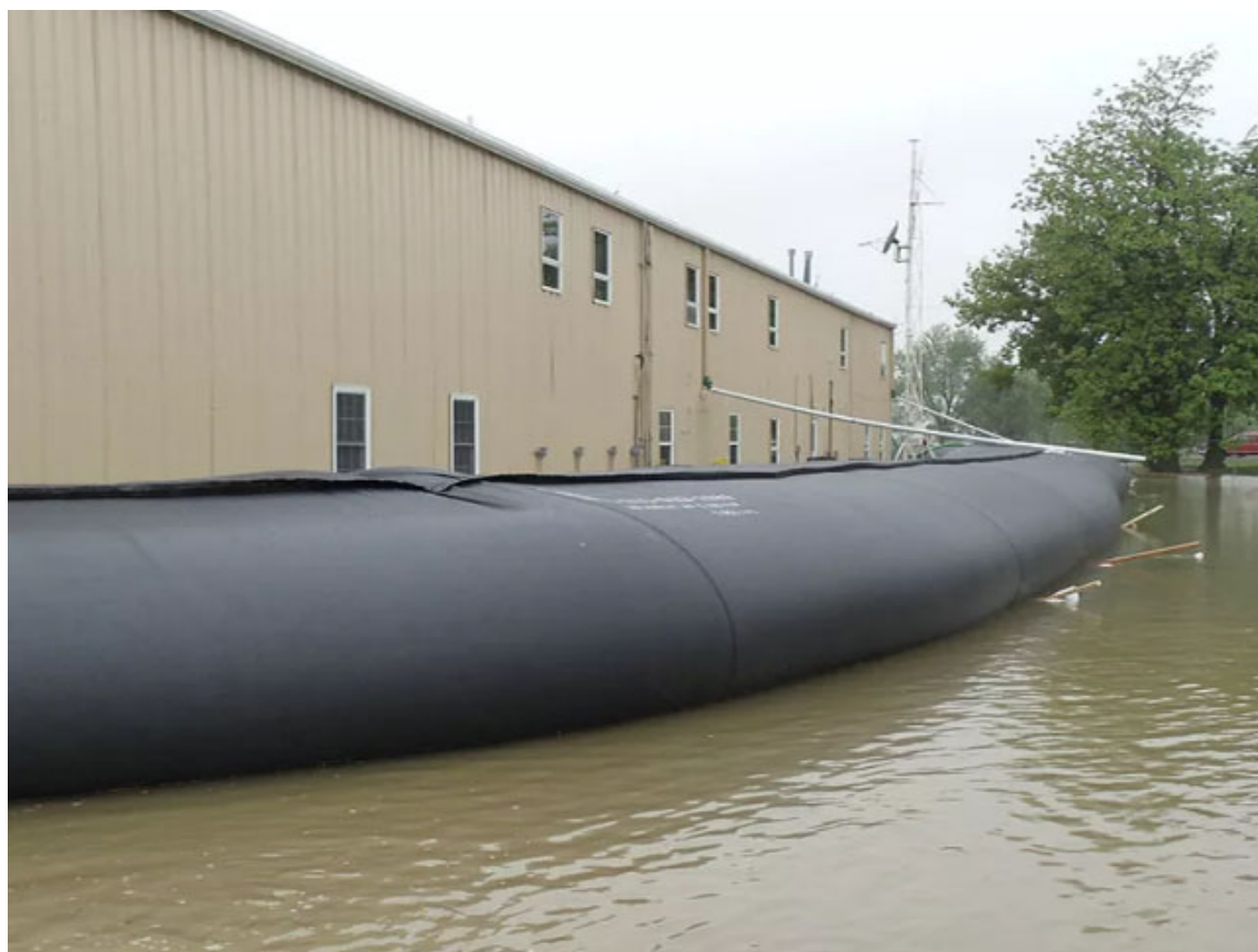
Water Filled Sandbag Equivalent Levee
