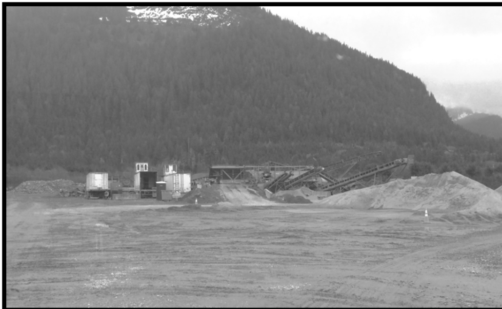
Figure 3: Rock crusher on Horecny Industrial Park site. Picture taken by CDD staff on 4/6/16
