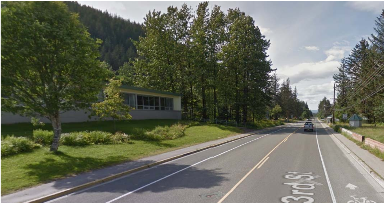
Looking north by Gastineau Elementary
