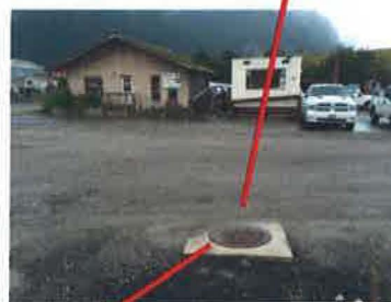
On site water shut-off About 12' deep
