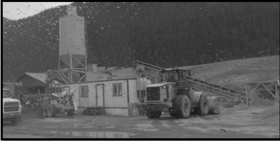
Figure 2: Concrete Plant on Lot 8A. Picture taken by CDD staff on 4/6/16.
