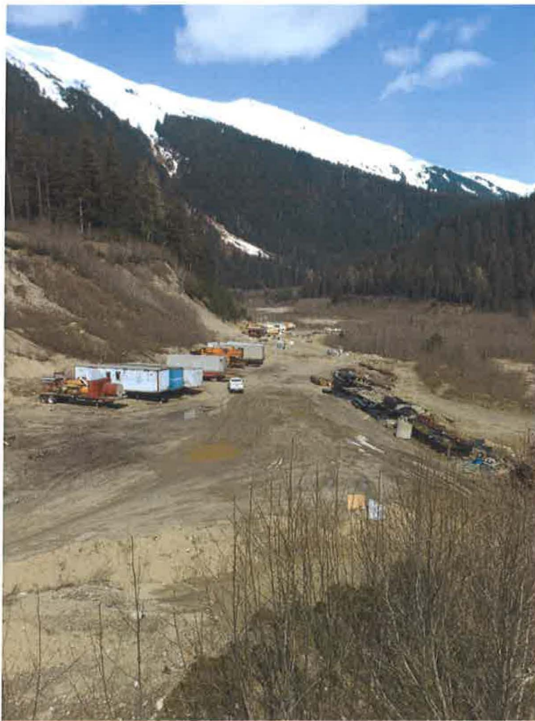
Image 18 - Hidden Valley Equipment Storage
