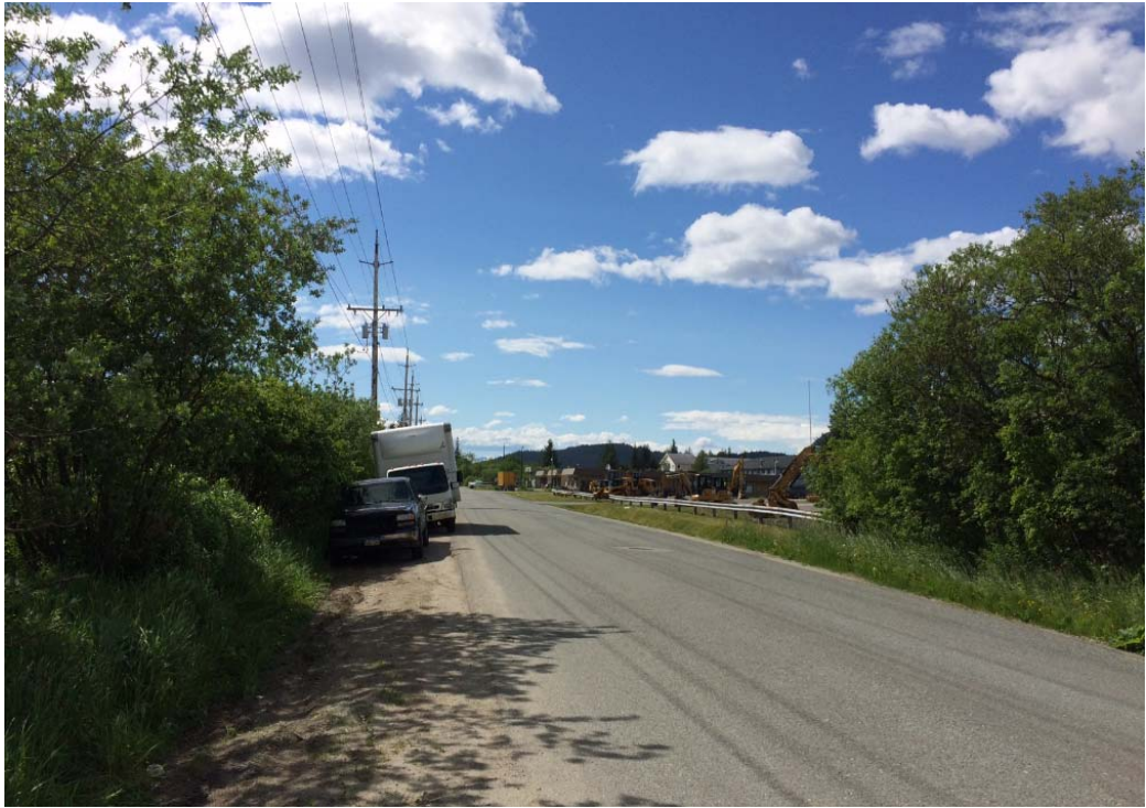
View West on Airport Blvd
