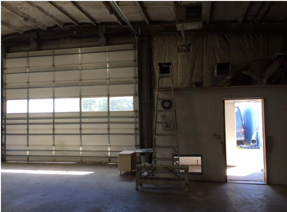
Inside view of Warehouse facing Entrance
