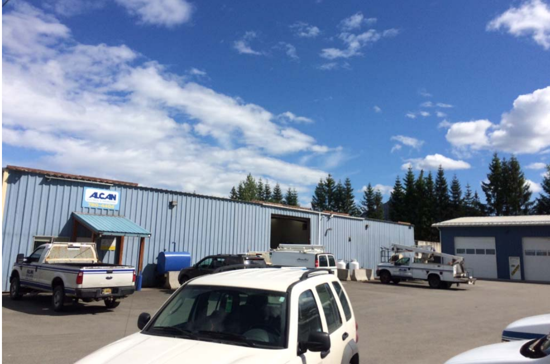
Subject Site and Parking facing south
