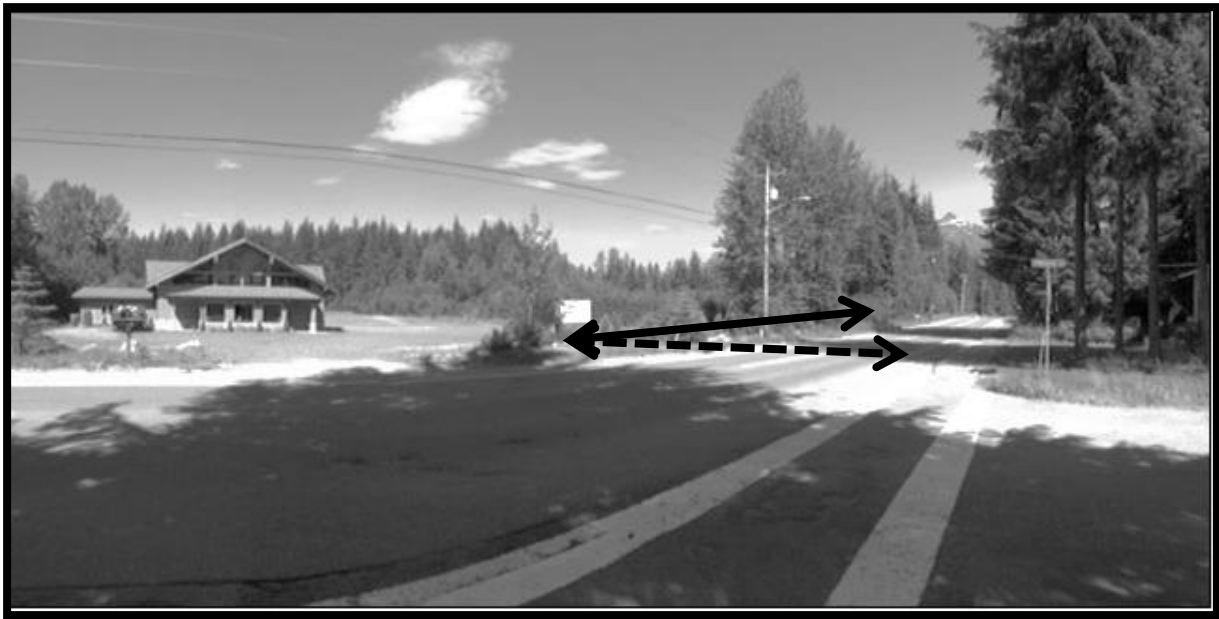
Figure 2. At the intersection of Pinedale St (Right) and Riverside Drive looking north. The Bethany Baptist Church is shown on the left. The solid arrow line represents the new sidewalk location and the dashed line represents the new crosswalk.
