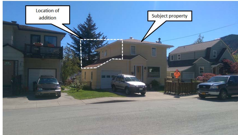
Attachment C: View of subject property from outside windows of 506 W. Ninth Street – additional will be constructed above garage
