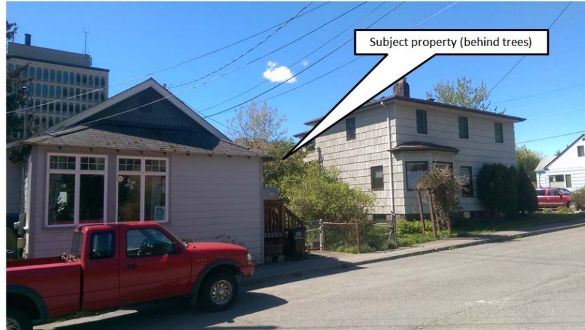
Attachment C: View of side subject property from outside of 815 ‘B’ Street – additional will be constructed above garage
