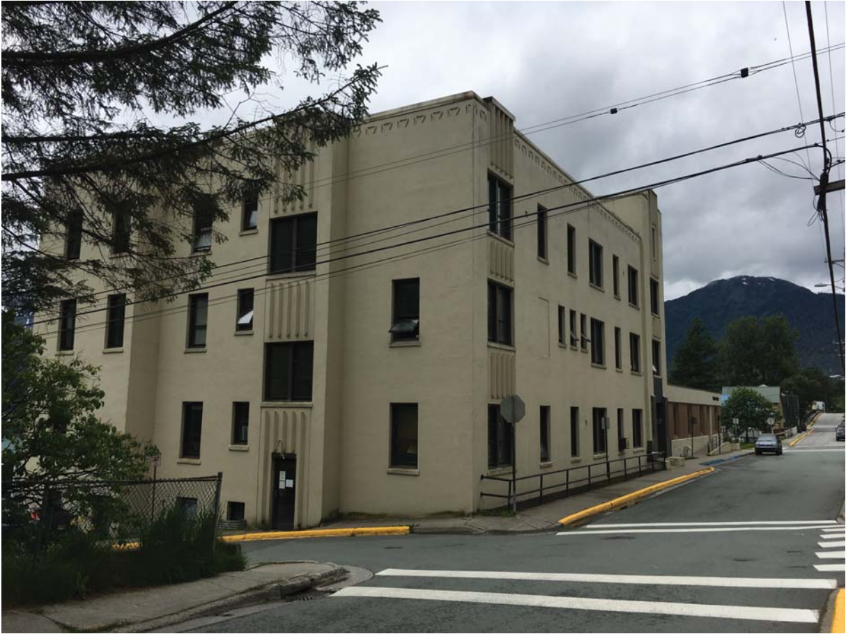
2017 - Catholic Community Services Building from Sixth and Harris Streets
