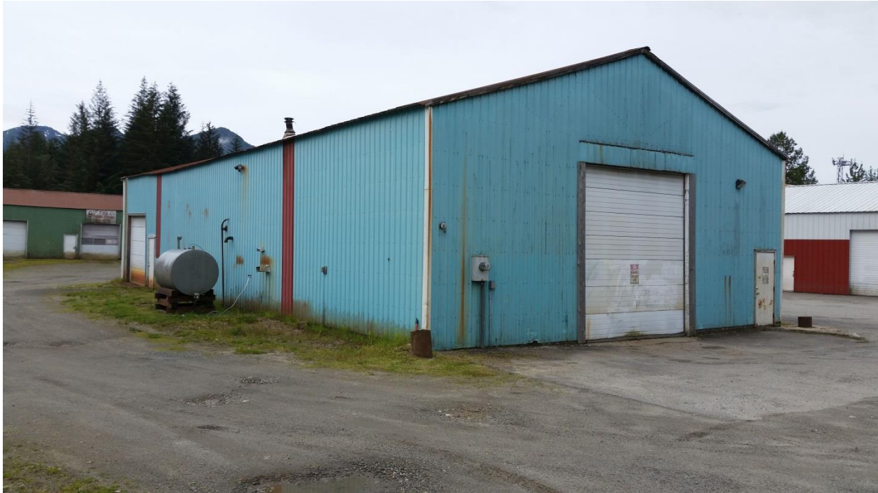
Figure 2: Unit A as seen from Jenkins Drive
