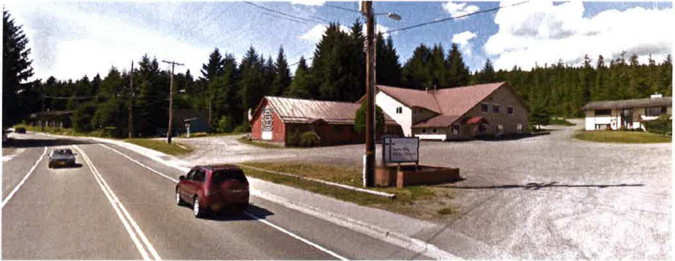
Fig 7: Road frontage, east to west view
