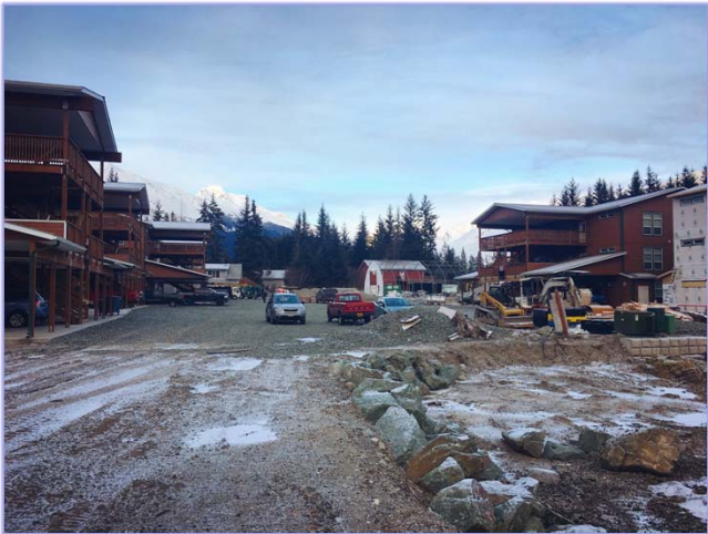
Recent progress Date: 01/10/18
