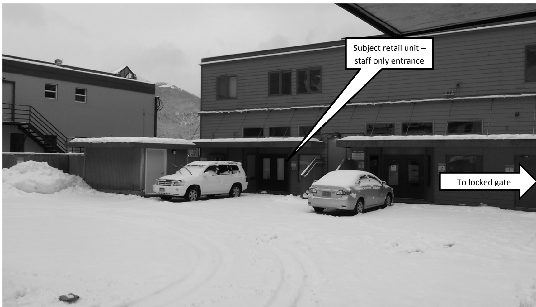
Attachment F: View of parking lot at rear
