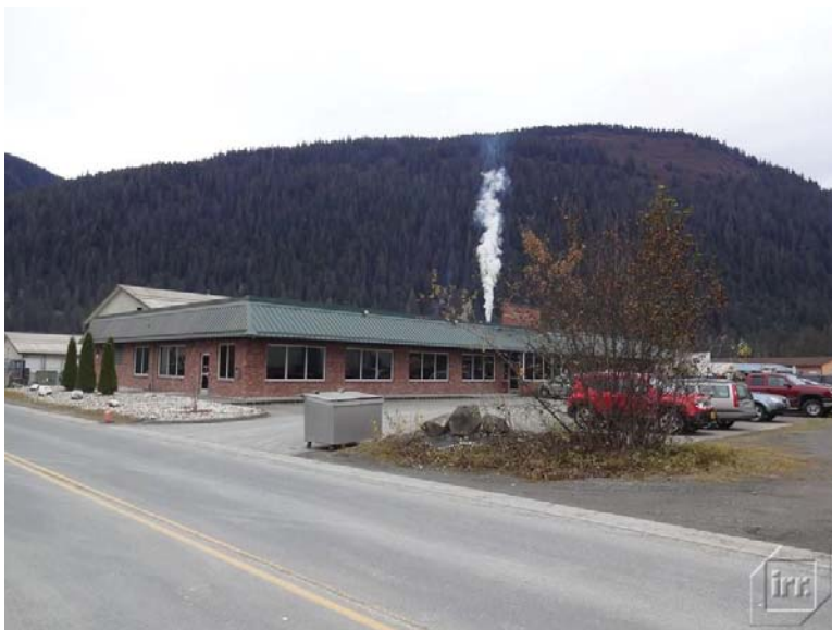
Vital Statistics Building 5441 Commercial Blvd Juneau, Alaska
