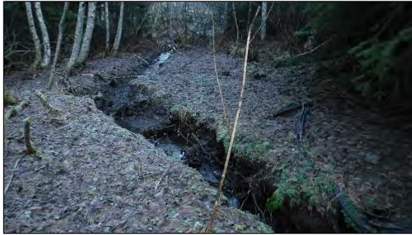
Figure 2.—Channel at toe of fill.
