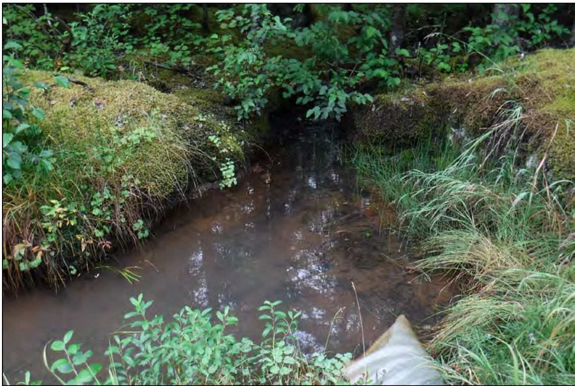
Figure 6.—Water from the ditch flows into Stream No. 111-50-10500-2015, cataloged for rearing coho salmon. View is looking upstream from culvert inlet.
