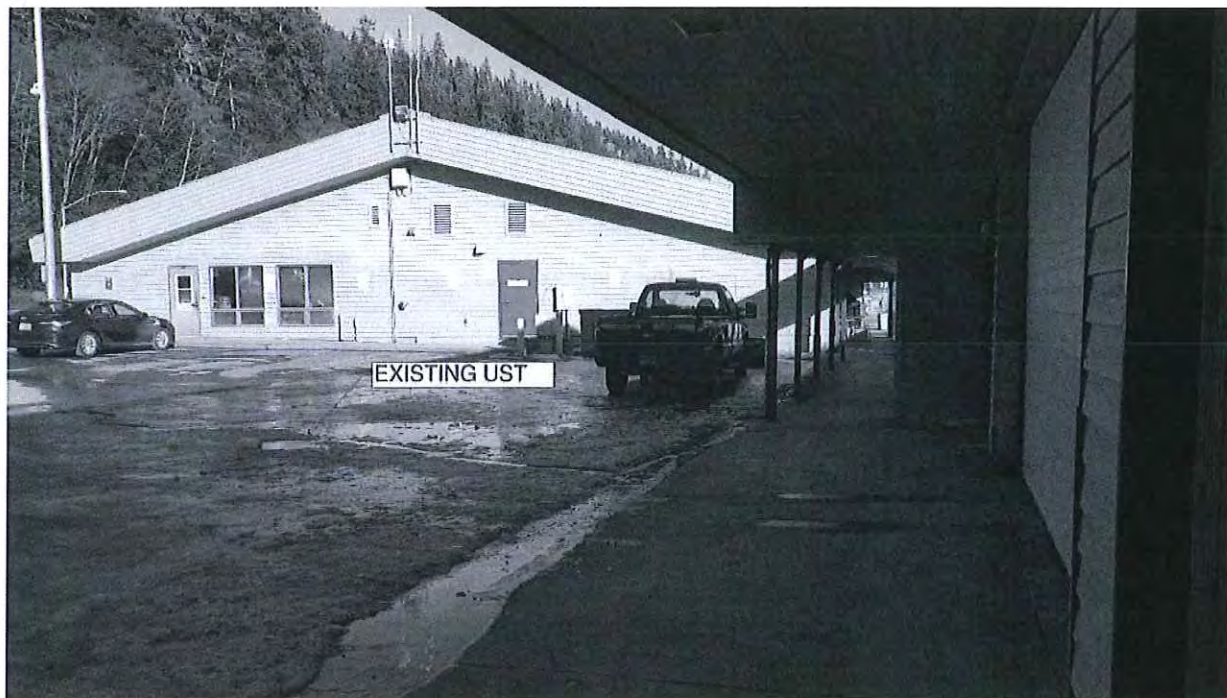
Figure 3: Fuel Tank Location in Auke Bay
