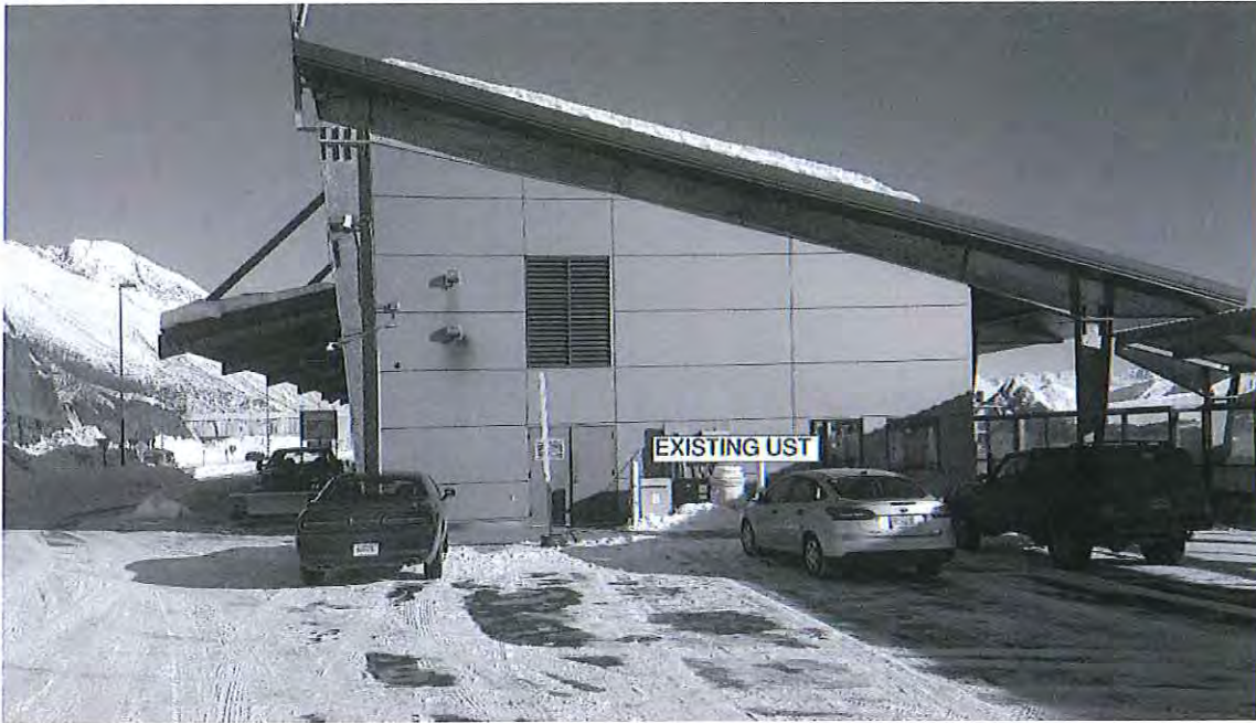
Figure 1: Fuel Tank Location in Valdez
