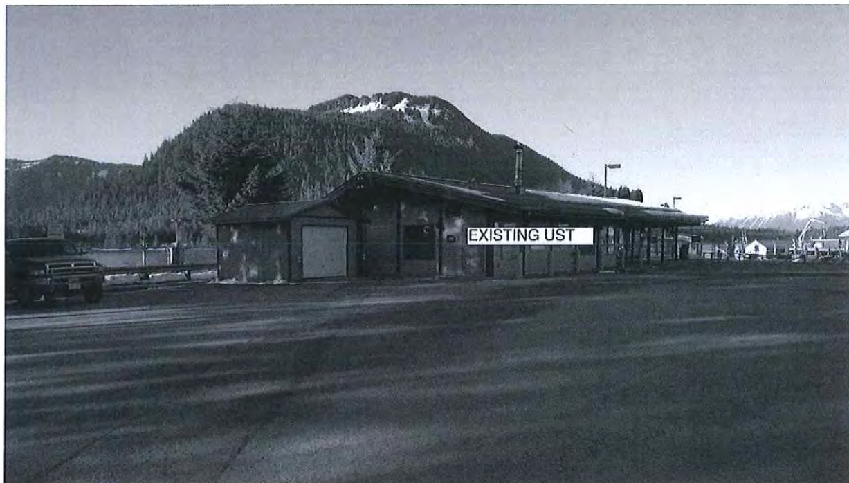
Figure 5: Fuel Tank Location in Petersburg
