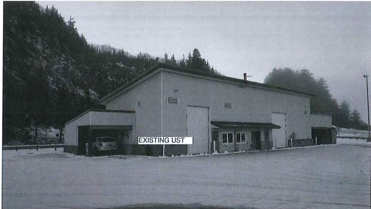
Figure 2: Fuel Tank Location in Cordova
