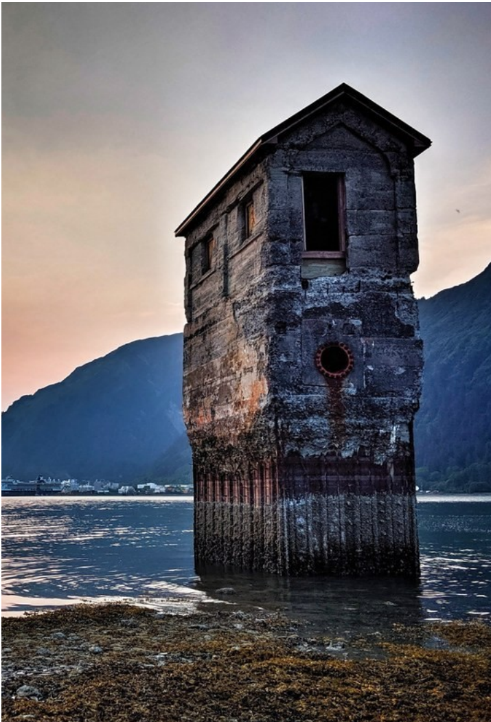
Old Treadwell Pumpphouse. Photo by Pat McGonegal.
