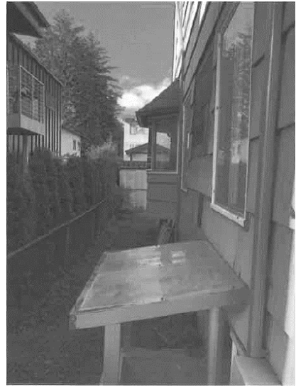
Photo showing an existing bay window (rear) and a structure protecting the basement egress window (foreground). The proposed chase will go behind the basement egress window, where some of the shingles have been removed.
