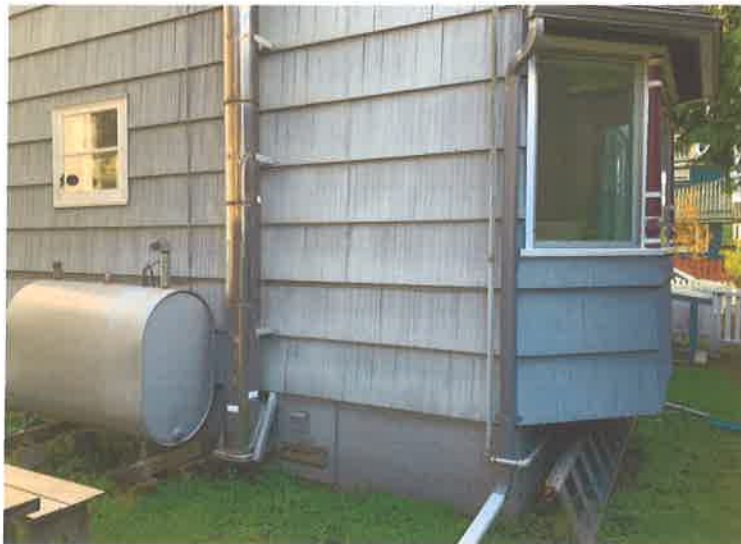
Rear of house - site of proposed propane tank
