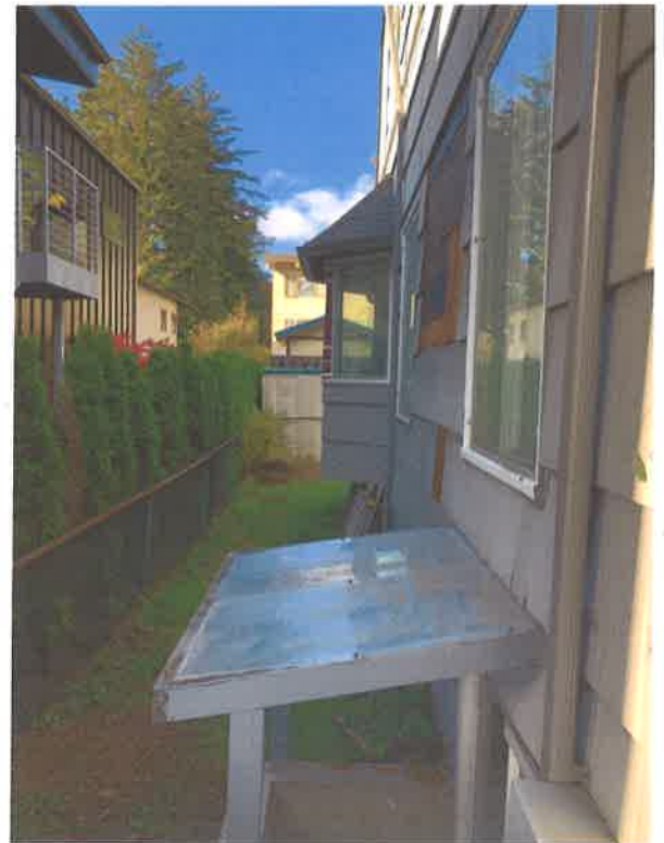
West side of house - ingress-egress window covering in foreground - foundation setback 7' 2" from fence (property line)
