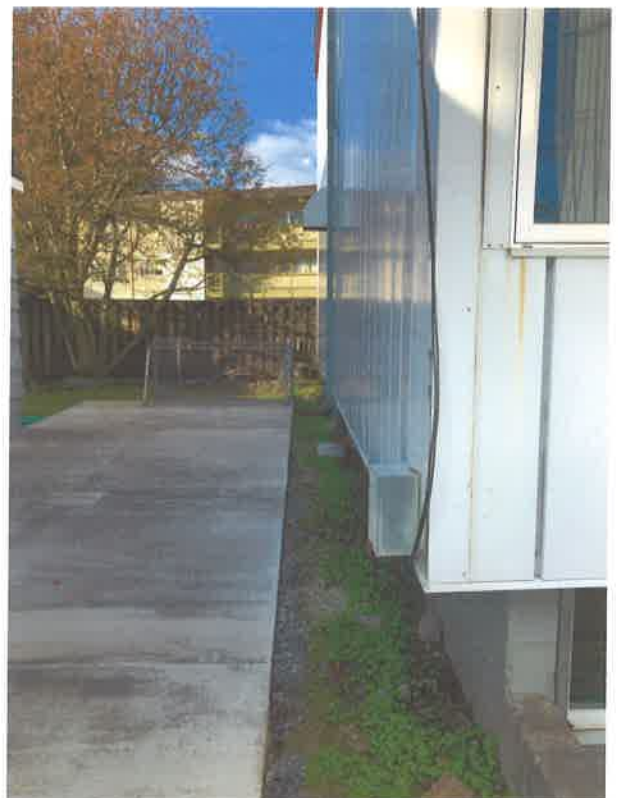
East side - Lot 12 - commercial offices with a basement apartment - wall is setback 23" from my driveway (property line)
