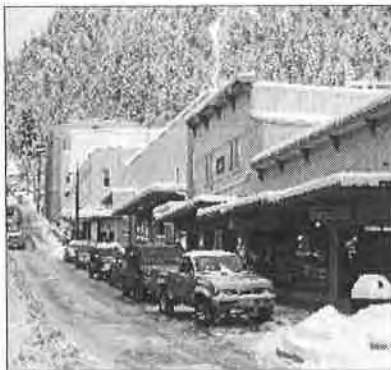
Canopies step with the street level.
