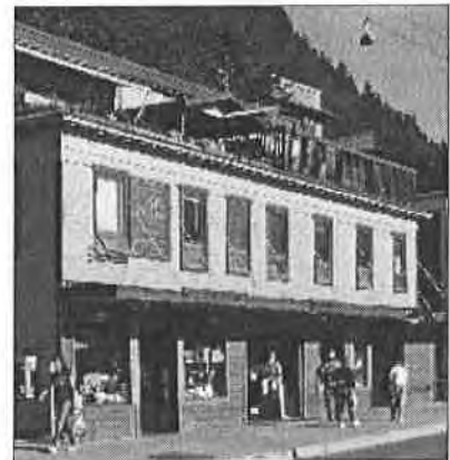
The rooftop use on the left side of the building includes an appropriately set back patio space. The rooftop use on the right includes a railing which is inappropriate and should be set back from the building facade.
