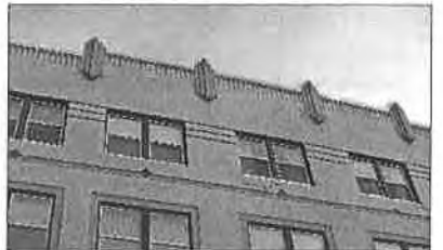
Cornice details in Juneau's Downtown Historic District.
