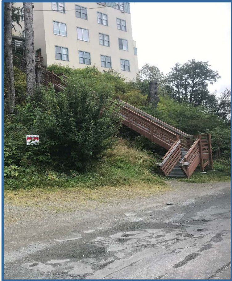
DISTIN AVE STAIRS
