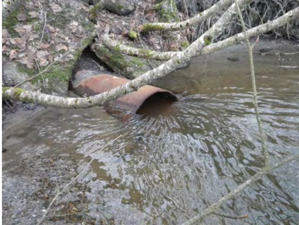
Figure 9. West berm culvert inlet at low tide.
