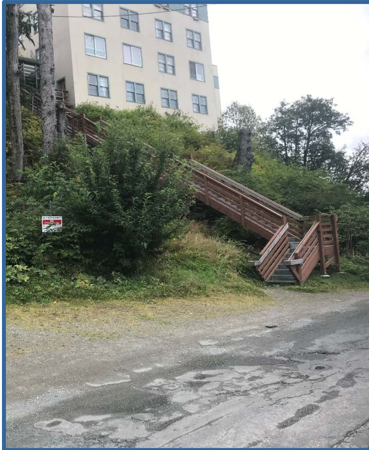
DISTIN AVE STAIRS
