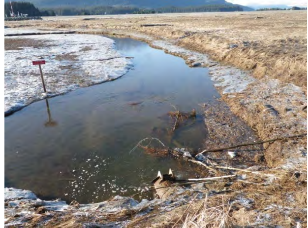
Figure 10. West berm culvert outlet at 1.8 m tide.
