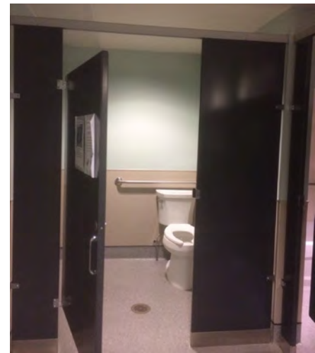
Figure 3: Example of accessible washroom, 3030 Gordon
