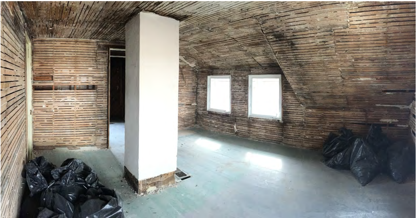
ABOVE: Top floor after plaster had been removed, exposing lathe.
