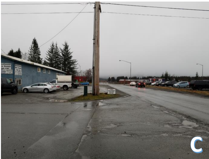
Picture C: Road at the south end of the project will slope to the west to mitigate drainage impacts to lower properties on the east, such as Southeast Mine Supply. Picture D: Muddy area used for parking around the Valley Lumber lumberyard driveway.
