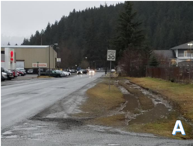
Picture A: Looking north from NC Machinery, the muddy ruts created by vehicle parking. Properties on the left use direct access to Crest Street from their parking lot (rather than using a driveway). Picture B: Looking south from Valley Lumber, poor ditch drainage on the right of a busy industrial route.
