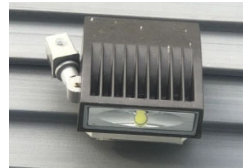
Existing exterior lights in situ
