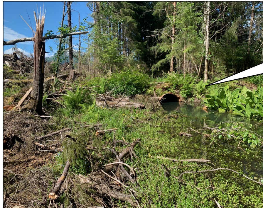
Culvert referenced in application
