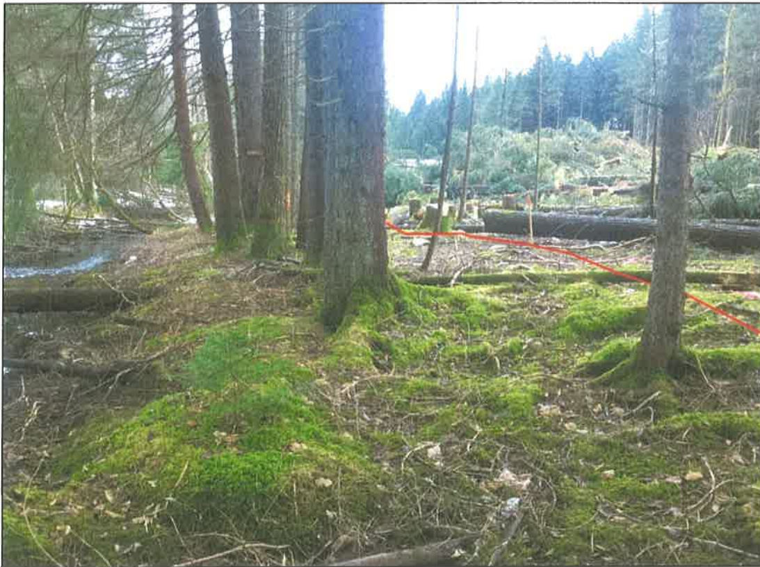
Figure 2.—Trees felled behind the proposed line staked in the field; Duck Creek on the left.
