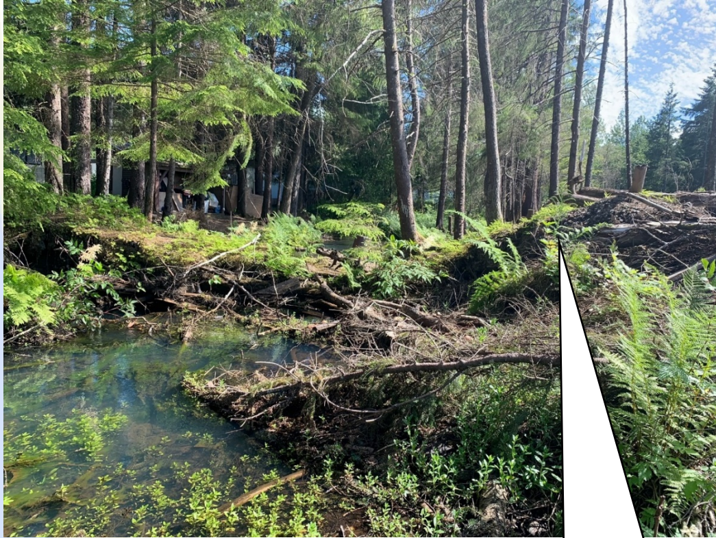
Collapsed log bridge referenced in application
