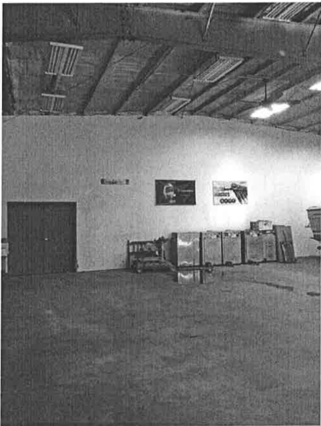
Inside view of Warehouse facing Alcan's portion of building
