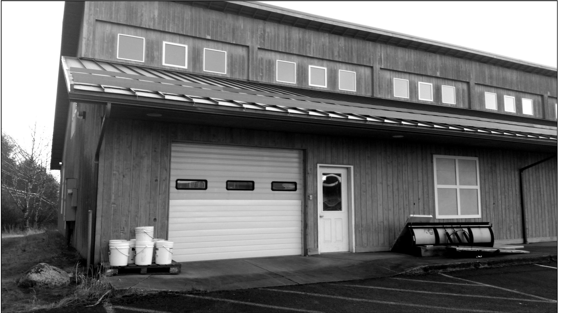
101 Mill Street, Loading Area
