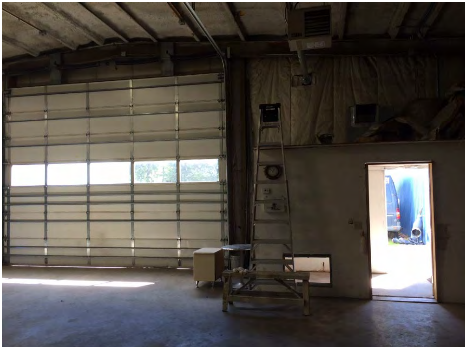
Inside view of Warehouse facing Entrance
