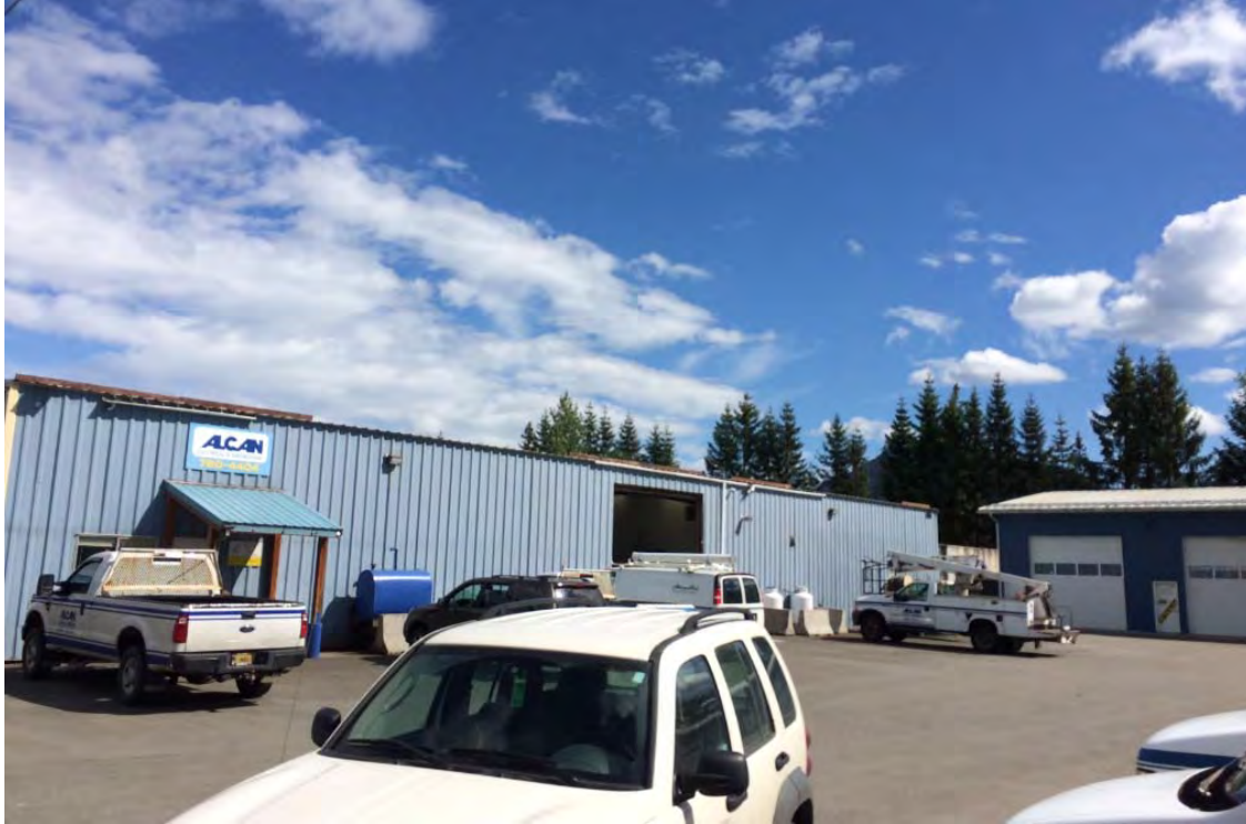
Subject Site and Parking facing south
