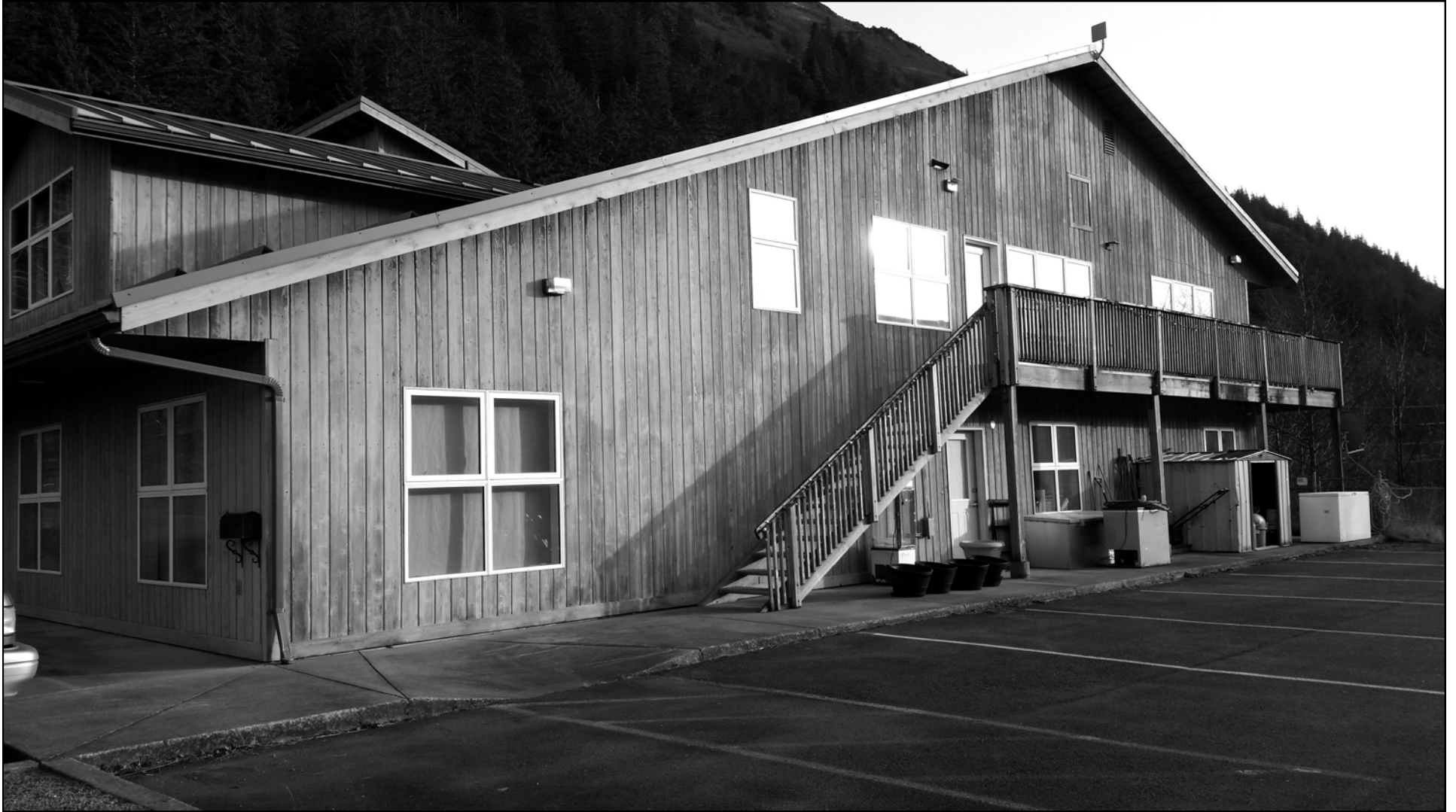
101 Mill Street, Retail Side
