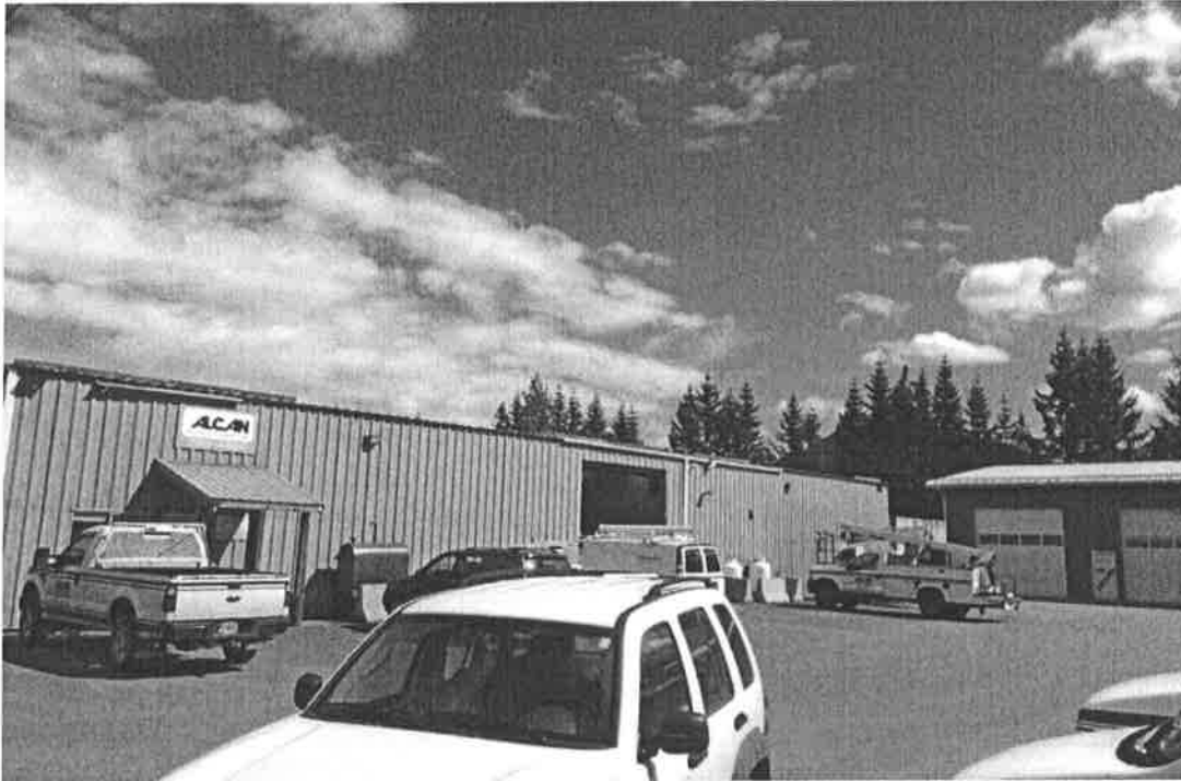
Subject Site and Parking facing south
