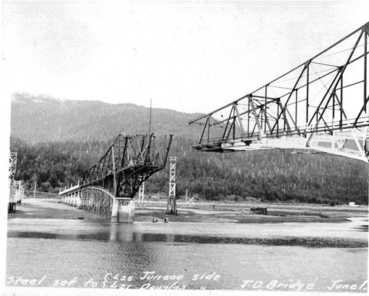
Juneau-Douglas Bridge Construction, circa 1935
