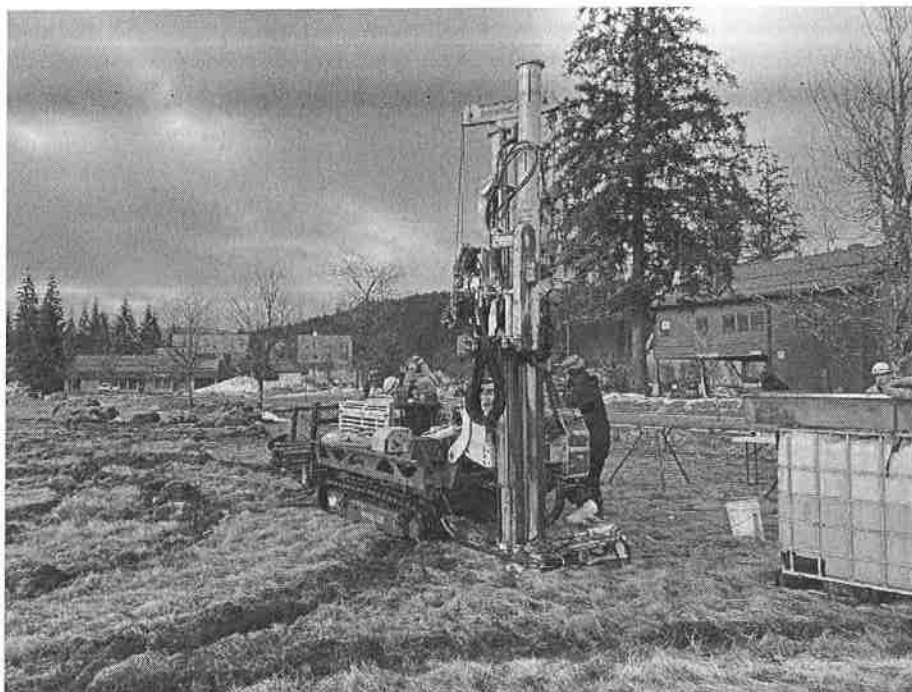
3. Boring at ENV-2 location
