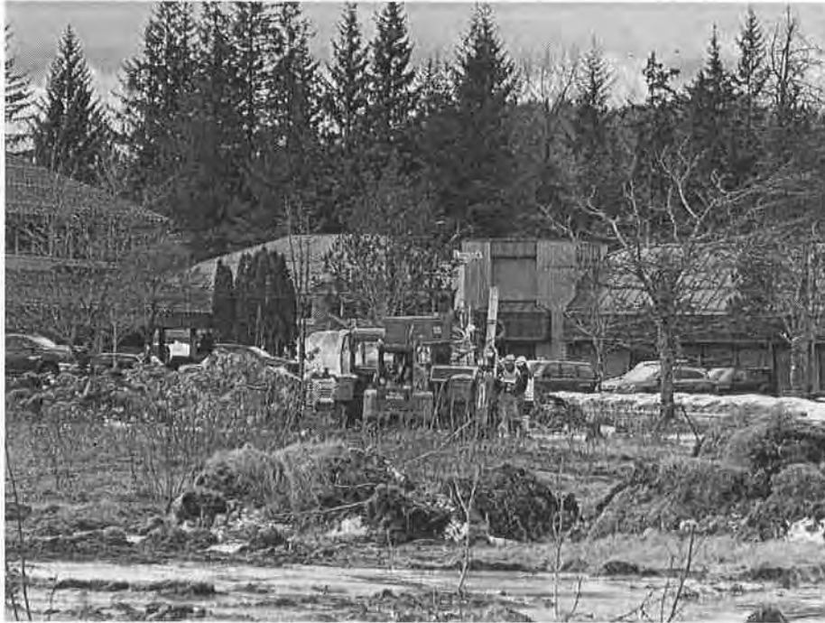
5. Boring at ENV-3 location
