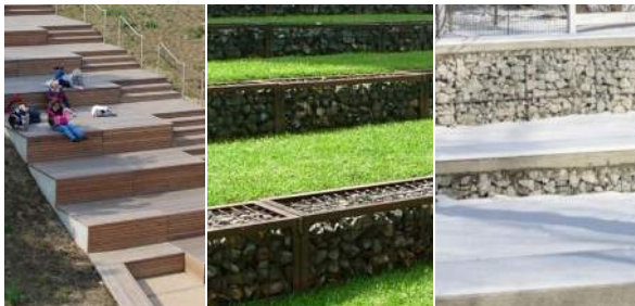
Gabion seat walls and stepped amphitheater
