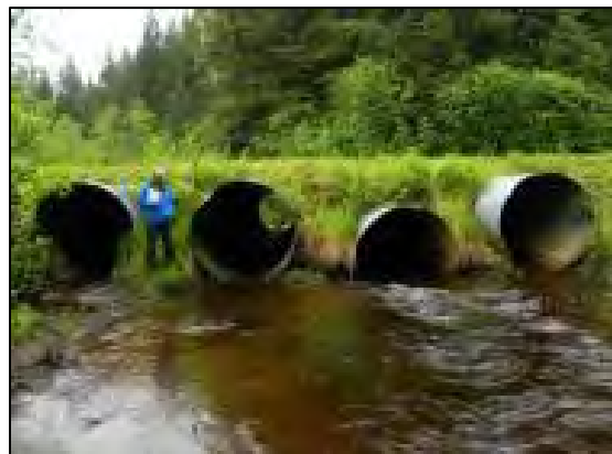
Figure 32. Four side-by-side culverts that create a low and high water velocity fish barrier on a side channel of Montana Creek. Photo courtesy of John Hudson, USFWS.
