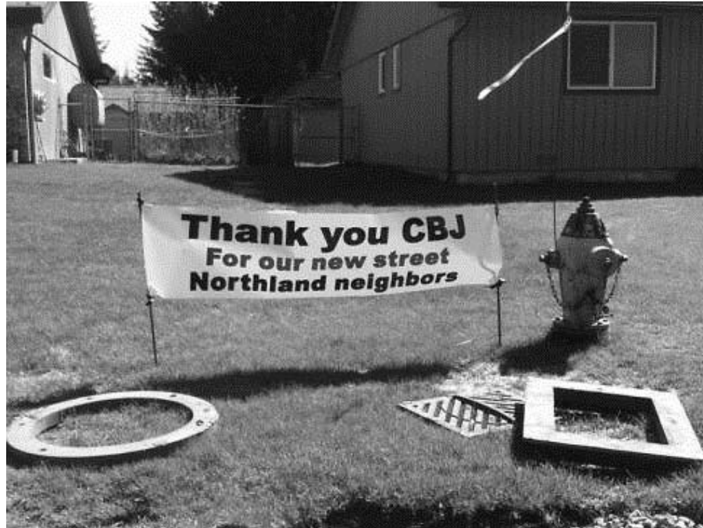
Northland Street Reconstruction
