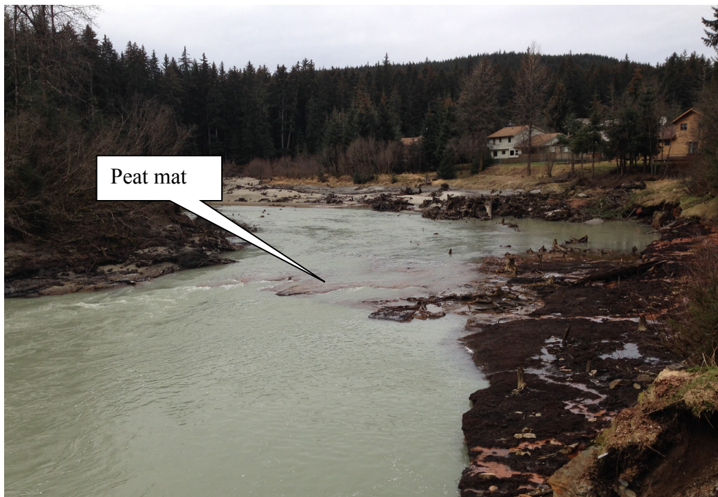
Figure 6: Peat mat at Meander Way bend of Mendenhall River
