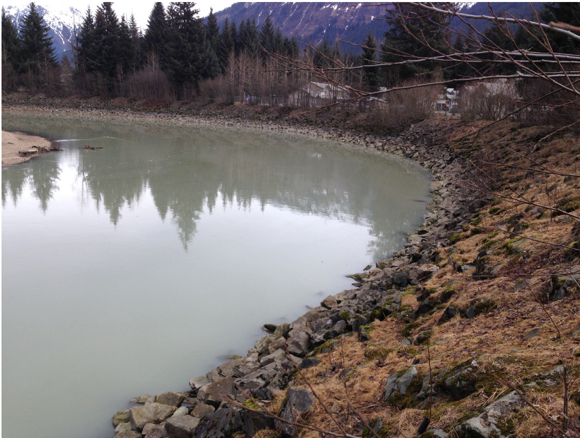
Figure 3: Existing riprap near Postal Way
