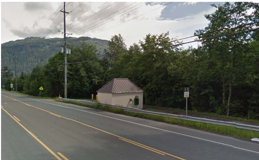
Gruening Park Pump Station Generator Building
