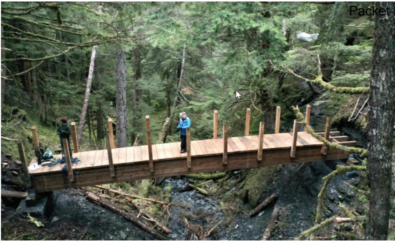
Treadwell Ditch Trail Renovation Project
