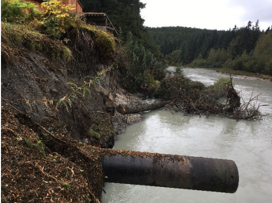
CBJ Rivercourt Way Storm drain outfall
