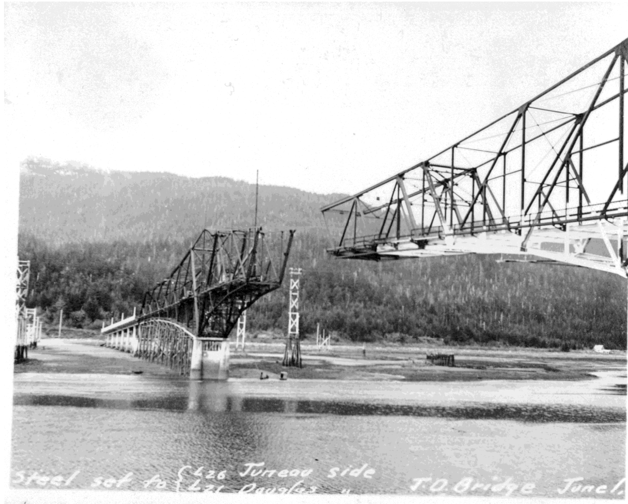
Juneau-Douglas Bridge Construction, circa 1935
