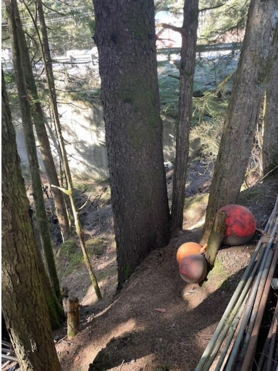
Looking north from the front of the property towards the Waydelich Creek bridge retaining wall.
