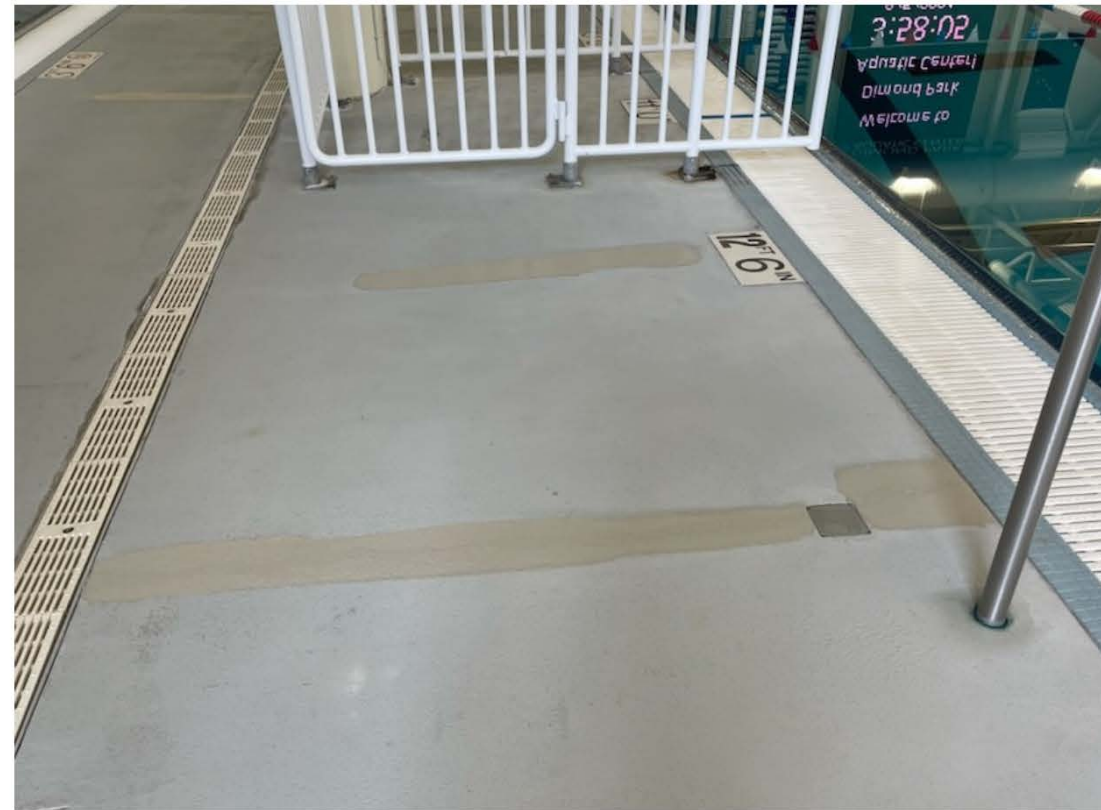
PHOTO AFTER REPAIRS.
