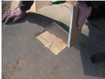
1/2" Rigid Insul under PVC Roof Membrane
