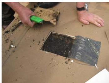
Built-up Asphalt Roof below OSB
