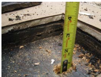
3/4" Plywood Roof Sheathing
