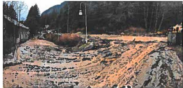
Mudslide and flooding at AWARE facility (Photo from http://www.ktoo.org )
