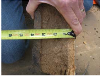
Low Roof Original Roof Assembly
