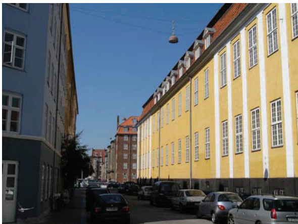
Figure 4 – Span-wire Overhead Light
