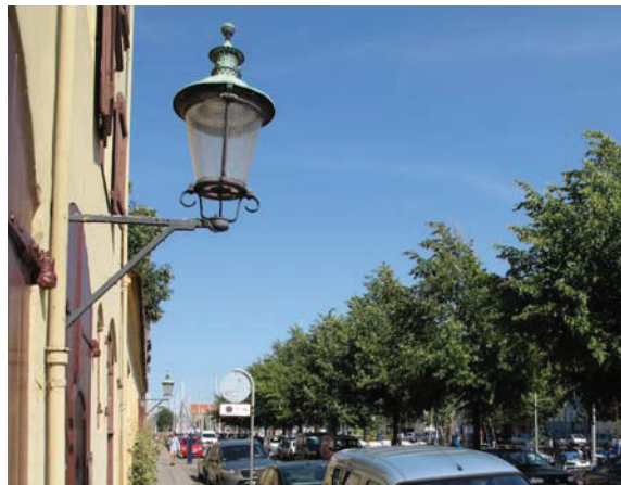
Figure 5 – Building Mounted Overhead Light
