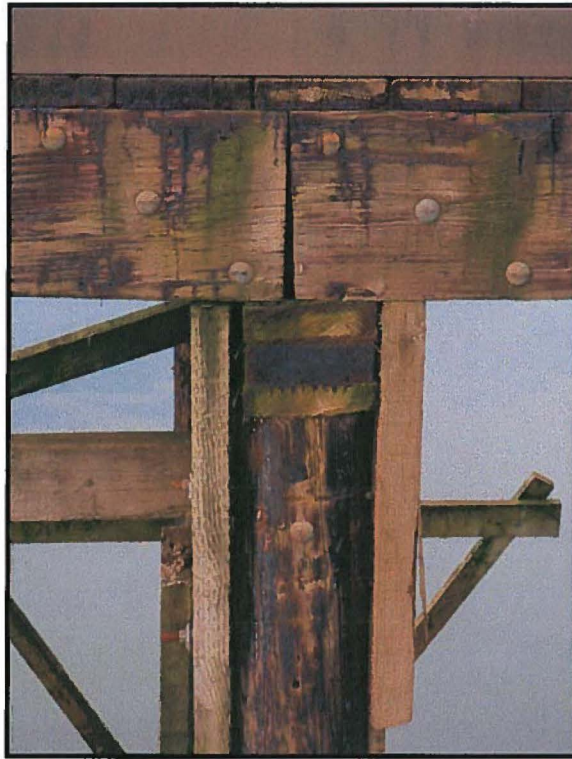
Supplemental stringer bearing detail.
