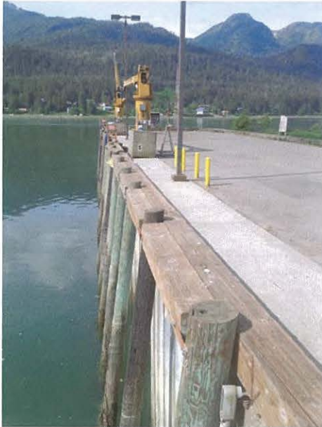
Detail of Fender Piles & Bull Rail
