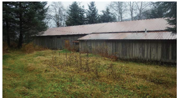
East side middle and south section
