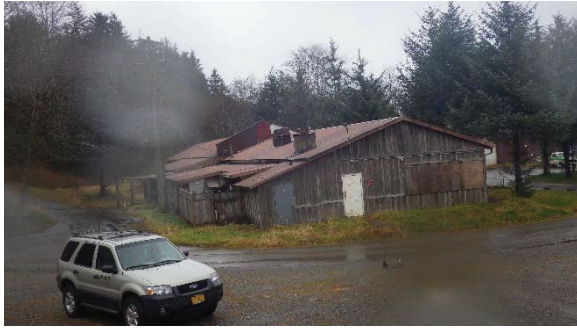
Thane Ore House from northeast
