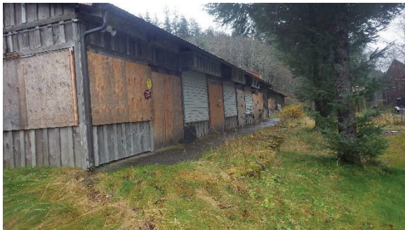
West wall from the north end
