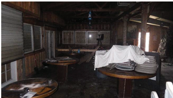
North section, west and north walls
