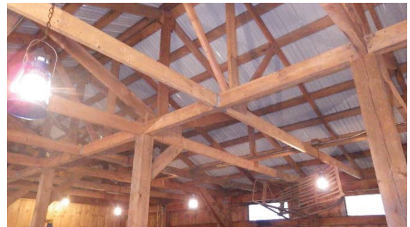
South section, intermediate trusses where double 2x6 support cuts through bottom chord
