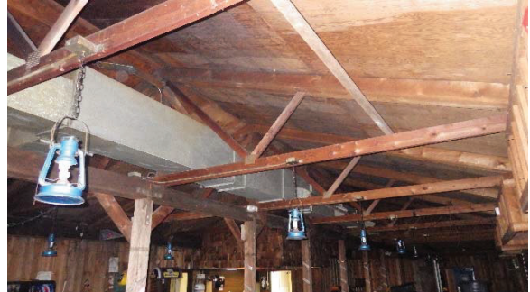
Roof trusses north section from northwest corner
