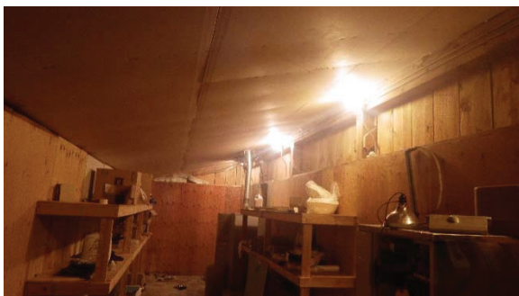
Storage Maintenance area middle section
