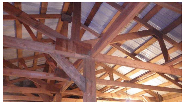
South section with truss on post with knee brace
