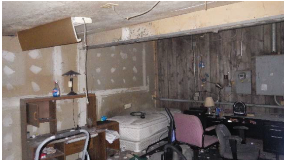
East side mechanical room with living quarters
