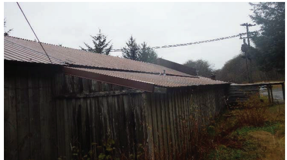
East side, middle section from south
