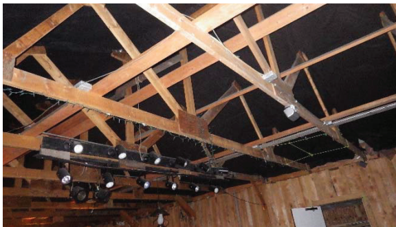
Middle section roof trusses
