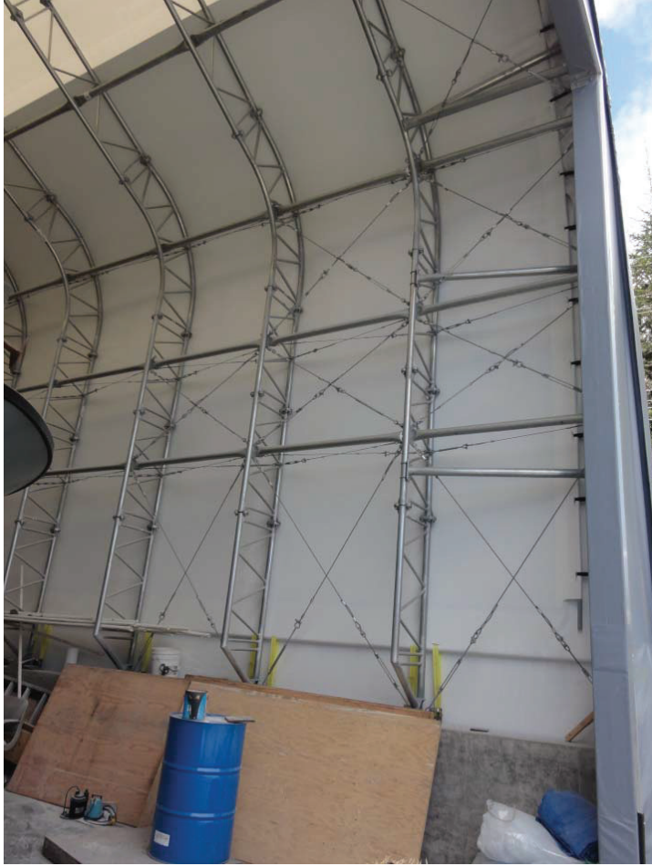
PHOTO 11 - INTERIOR OF FABRIC BUILDING. NOTE THE HIGH CONCRETE SIDES AND THE TIE DOWN STRAPS CONNECTING THE FRAME TO THE CONCRETE SLAB. 051518_2555)
