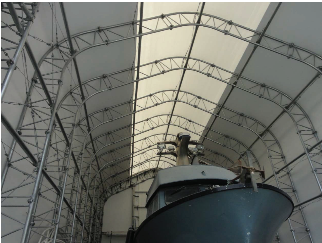
PHOTO 10 - LOOKING INTO FABRIC BUILDING (051518_2556)
