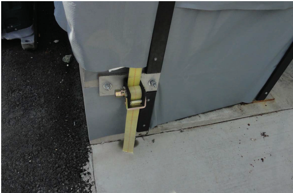
PHOTO 12 - CONCRETE FOUNDATION WITH TIE DOWN STRAP AND FABRICATED BUILDING FABRIC. (051518_2554)
