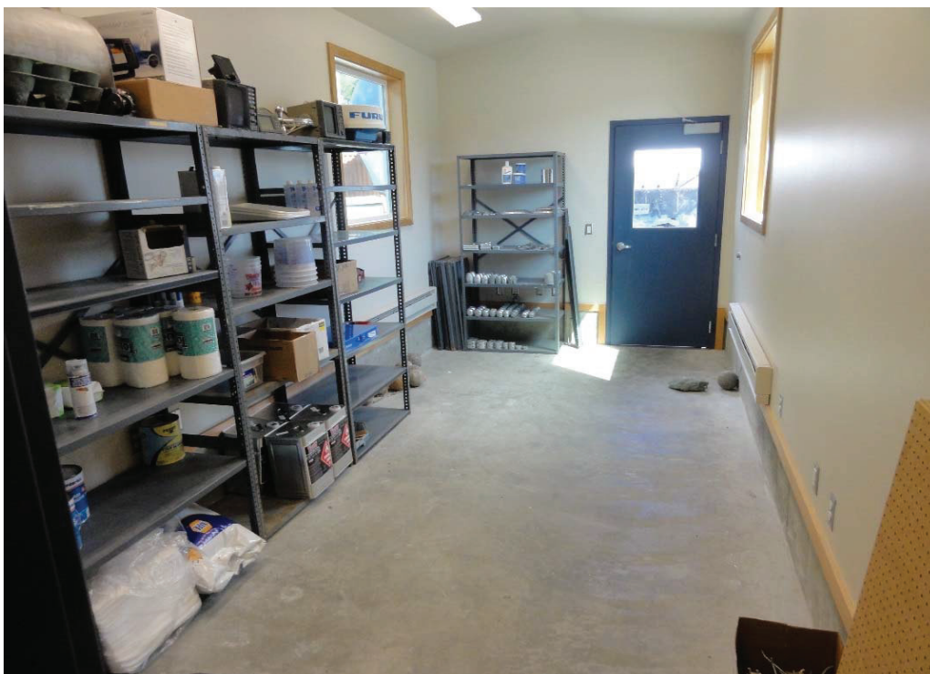
PHOTO 8 - INTERIOR LOOKING FROM EXISTING BUILDING INTO ADDITION. (051518_2541)
