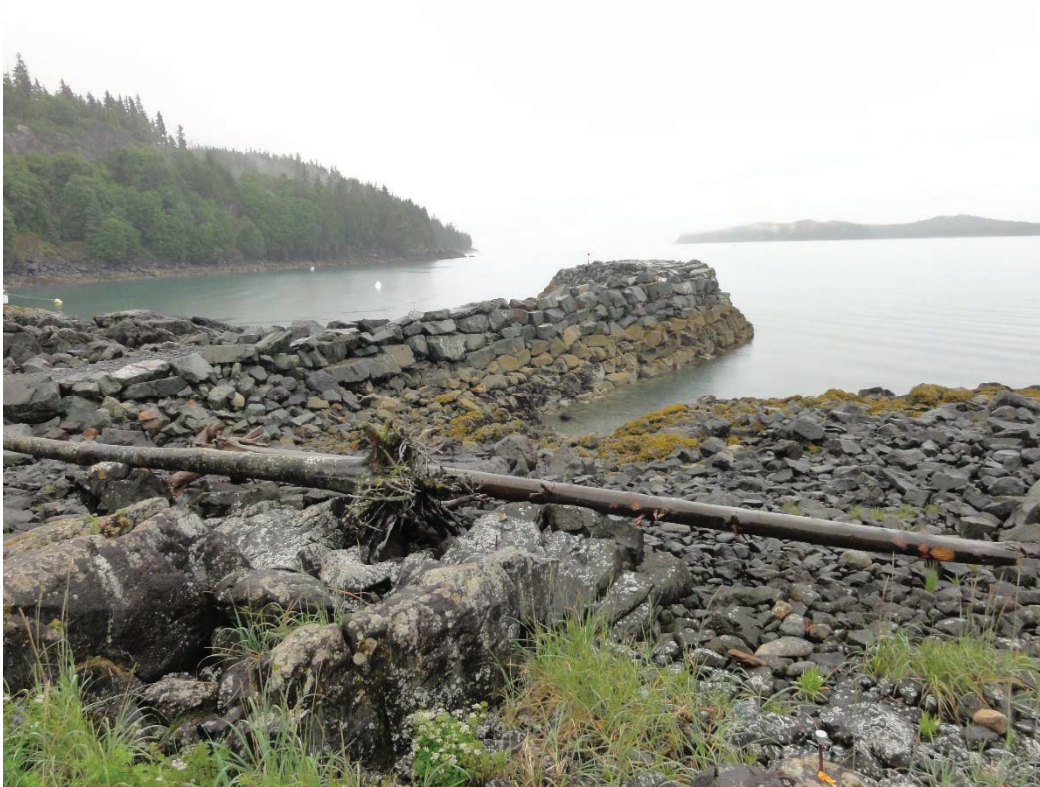
PHOTO 8 – LOOKING SOUTH AT WESTERLY SIDE OF BREAKWATER. (071317_0877)
