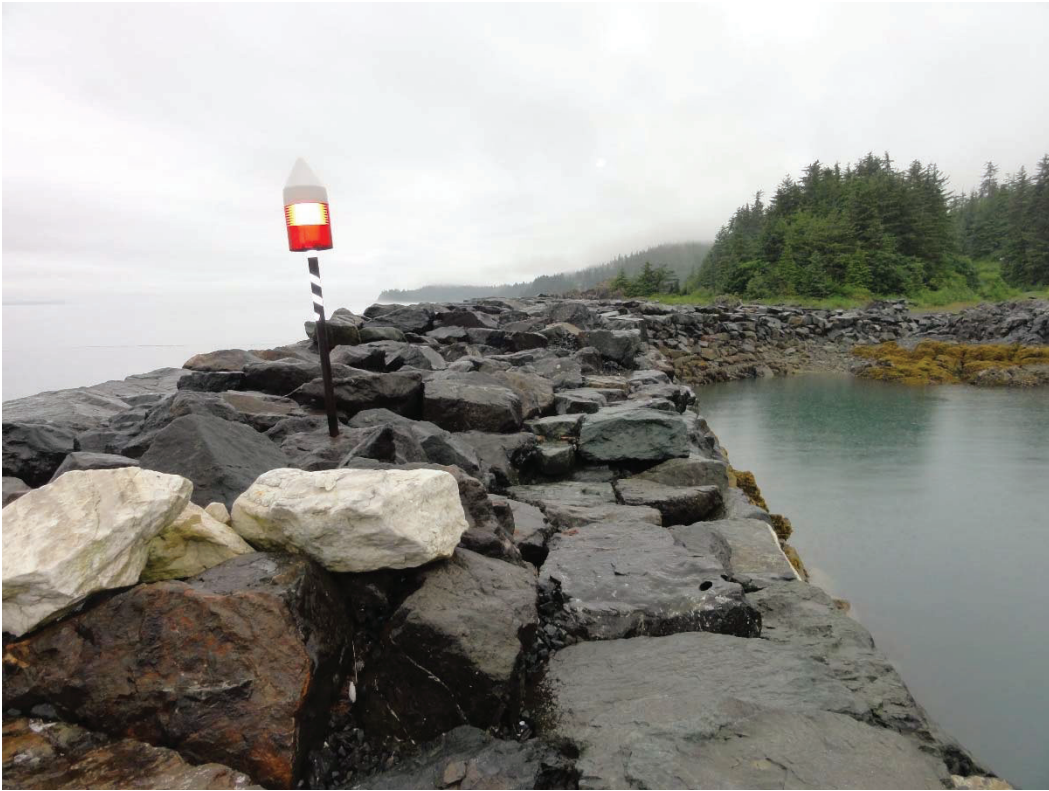
PHOTO 7 – LOOKING NORTH FROM END OF SUBJECT BREAKWATER. (071317_0874)
