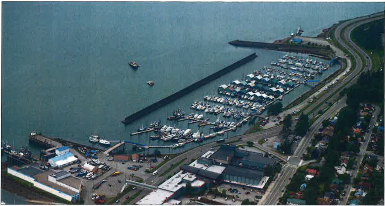
Figure 6. Aerial view of Aurora Harbor, Juneau (USACE 2017).
